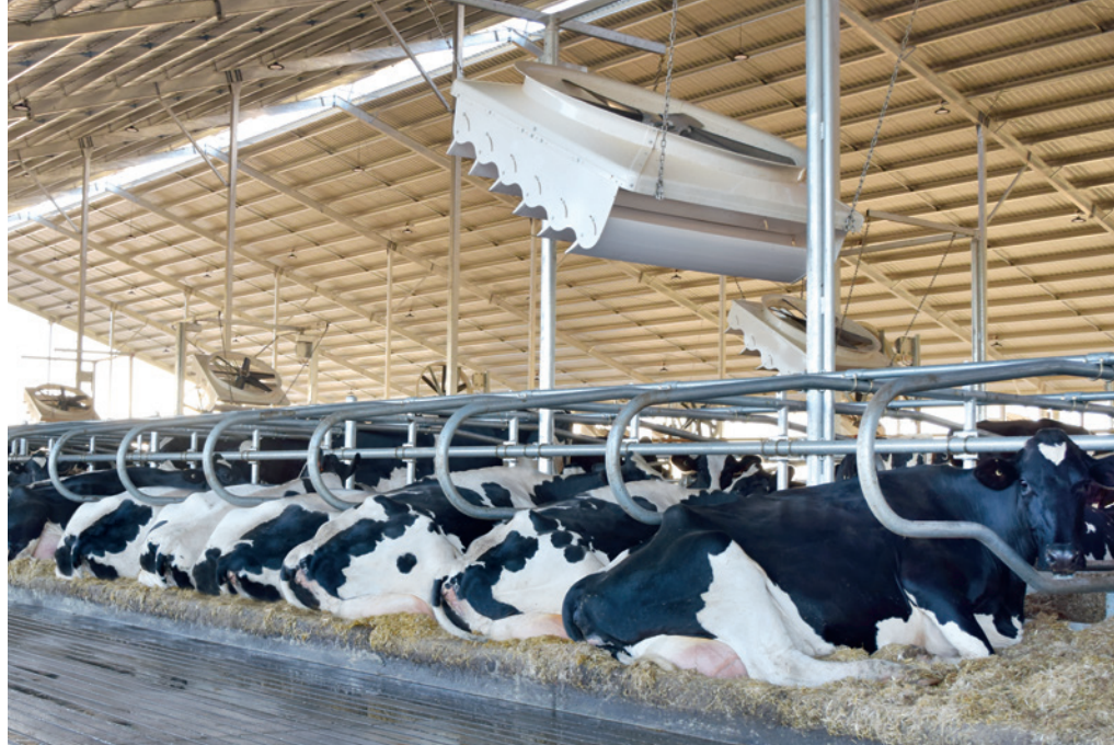
The cows are achieving 14-15 hours rest a day in this facility.
