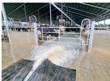
Ray Smith chose to use fresh water for the flood-wash because it keeps the facility cleaner, and it isn't wasted.
