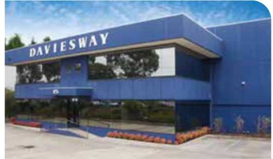
Daviesway and DASCO’s head offices sit adjacent to one another in Melbourne.
